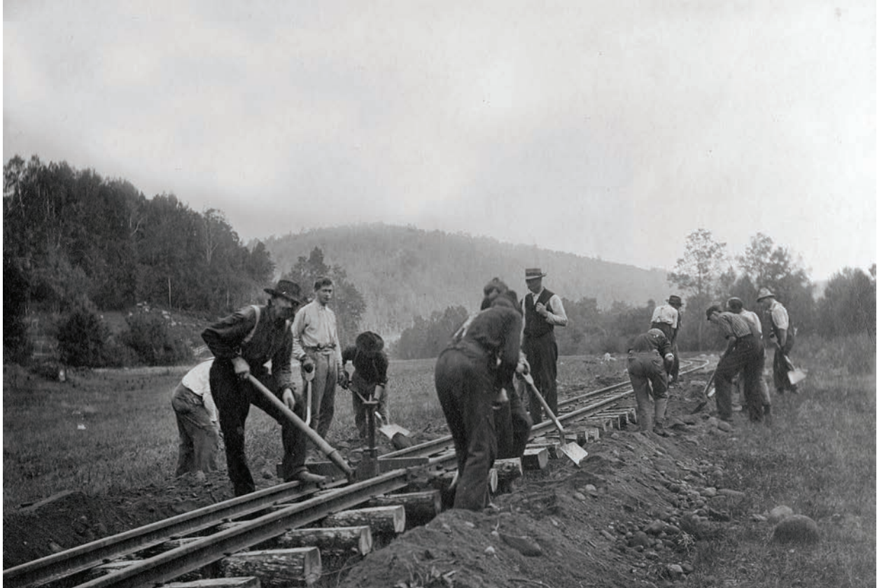
A photo of the 1910 Madrid extension and the ballast crew using a jack and level in the gauge to raise the rails when leveling the track for use. Six men in this photo can be identified in the group photo on the flatcar. F.A. Lawton is the person standing in the gauge. (Courtesy of Phillips Historical Society, Phillips, Maine)
