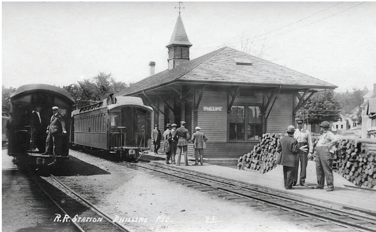
Phillips station after automatic couplers and air brakes were added to the passenger cars. At this time the platform extended beyond the station between the mainline and the Dana track, with a sand pile being used as a bumper. This was later replaced with a proper bumper as seen in later photos. The name Dana track comes from Elliott Steward and his book Sunset on the Sandy River . The piled wood waiting to be loaded is peeled pulp. (Author's Collection)
