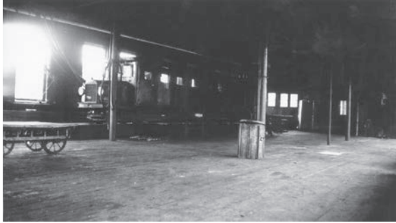
An interior view of the carpenter shop at the end of operations with the railbus. (Author's Collection)
