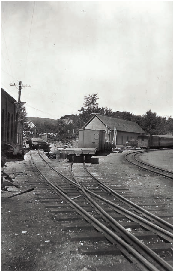
Phillips yard in July or August 1909. Construction of the new shop building was underway after a building referred to as the carpenter shop had been torn down. On the left-hand side of the photo are the rear windows of the enginehouse that were bricked in, which we will read about much later. The two flatcars and the boxcar seen here are further examples of no numbers or visible report markings. The building on the right is the last car house built, which was torn down in April 1910. The caboose is the No.553 and next to it on the ground is a locomotive cab, showing us that even though new shops were under construction, locomotive overhauls continued. It is unknown which locomotive the cab belonged to or where it was being rebuilt. (Courtesy of Walker Transportation Collection, Beverly Historical Society, Beverly, Massachusetts)
