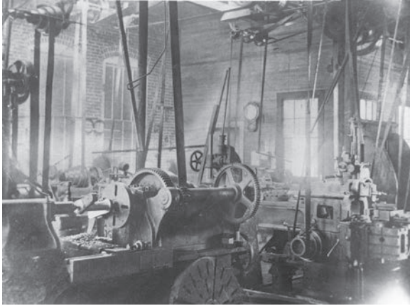
A Phillips machine shop photo that predates December 1922, when the skylights were removed and a cupola was added. This photo gives a good example of how much sunlight the skylights allowed in. The shop machinery shown here was driven by the overhead belts and pulleys.
