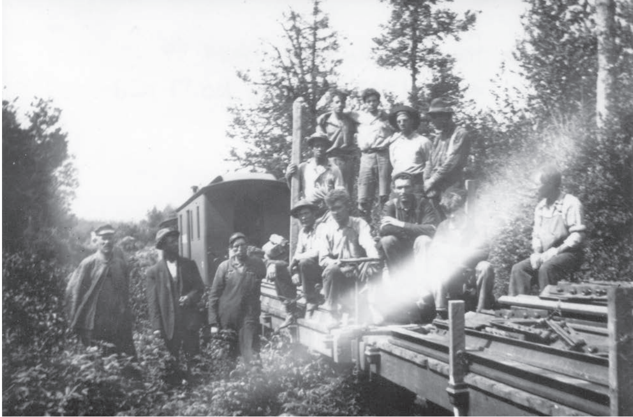
Baggage car No.5, with the opposite side seen than in the previous Greene's Farm photo. It is believed to have been taken later the same day, southward between the Skunk Brook Branch and the former Berlin Mills camp. On the flatcars are examples of how Sandy River & Rangeley Lakes scrapping crews left nothing usable behind, including tie spikes. Here we have a clearer view of the side of No.5 showing large white block lettering between the baggage doors, similar to the earlier photo at the International Mfg. Mill at Phillips, which was only a few months after this photo. In the lower corner is a blurred car number. I bring this up only because records claim it was renumbered No.7 in 1910. (Courtesy of the Phillips Historical Society, Phillips, Maine)
