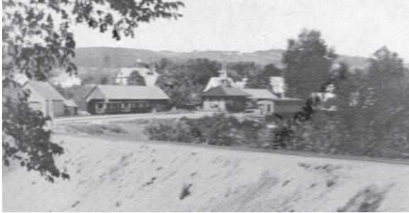
This photo is noted as 1902, and the two excursion cars are next to the car shop that was torn down in 1909. The white building on the left was the original Sandy River railroad car shop. Both buildings are covered in The Next Stop is Phillips . (Author's Collection)
