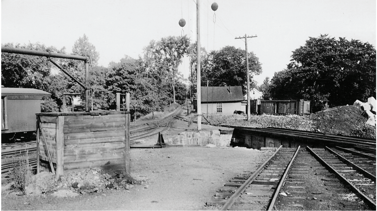
Looking south towards Farmington. On the left is the Phillips watercrane shown years after the 1908 article. In a later 1910 yard photo, you can compare the watercrane changes over the years. This ball signal seen here controlled movement into the yard, and is referred to in later photos as semaphores/signals become a more prominent subject. The steel turntable seen here was installed in 1921. The boxcar in the background is on the Braymen spur. (Author's Collection)
