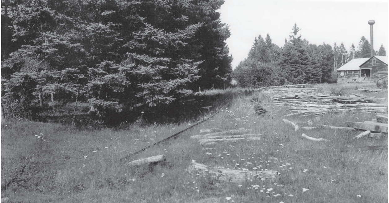
The Savage Mill, which is one of only a few photos of any mill at this location. In the foreground a few rail strings are on their sides in the weeds. In the distance, the light opening through the trees is the field and 1917 location of pulp loading operations. When pulp at Greene's Farm and Langtown operations ceased, so did all business on the former Eustis railroad. (Author's Collection)
