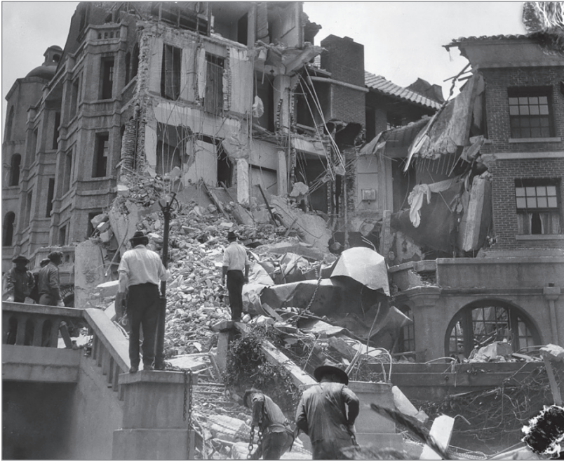
Buildings damaged by the Long Beach 1933 earthquake
